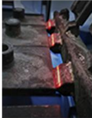
Laser to signal the cut site.
